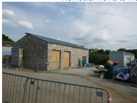
New Energy Centre
