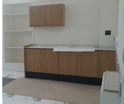
2 nd Floor Classroom Wet Area
