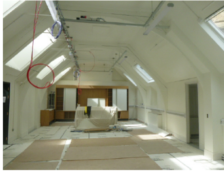
2 nd Floor Classroom
