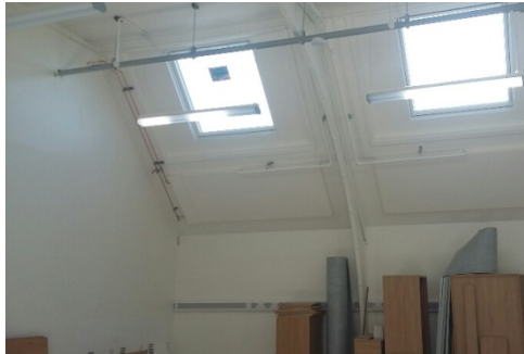
Replacement velux windows installed
