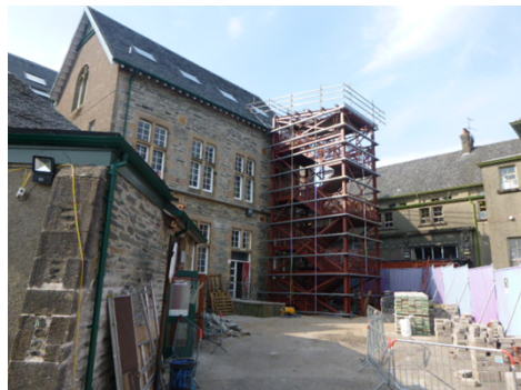
Temporary Escape Stair Installation
