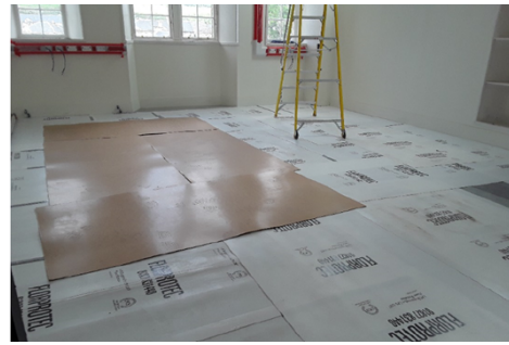
Protective covering to new flooring
