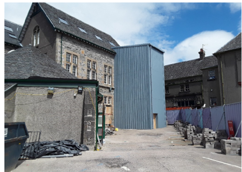
Complete Temporary Escape Stair
